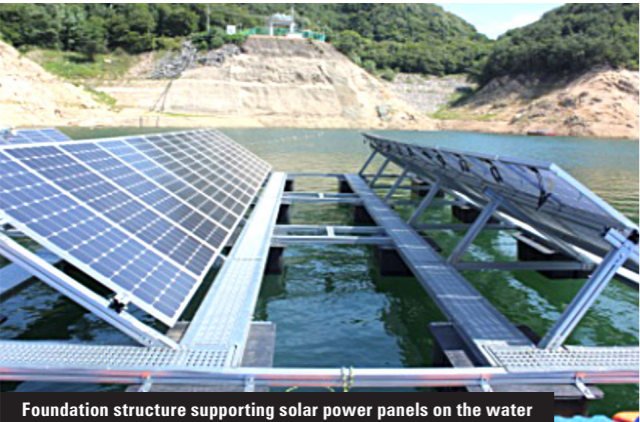
Foundation structure supporting solar power panels on the water
